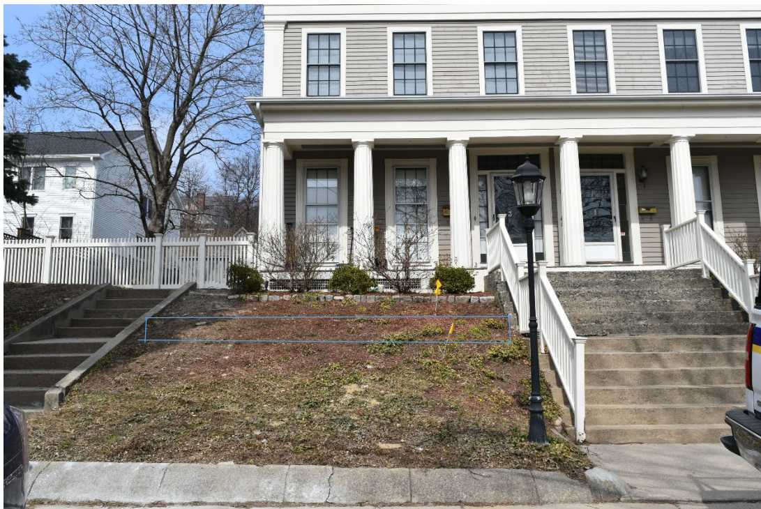
Garden Stairs (left) and Main stairs (right). Existing slope soils are sluffing and eroding downhill. The blue line shows the mid-level wall which will reduce the angle of the slope uphill. Downhill slope and groundcover will be left largely intact.
