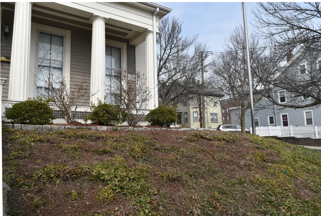
Detail image of the top of slope showing pocketing and erosion.
