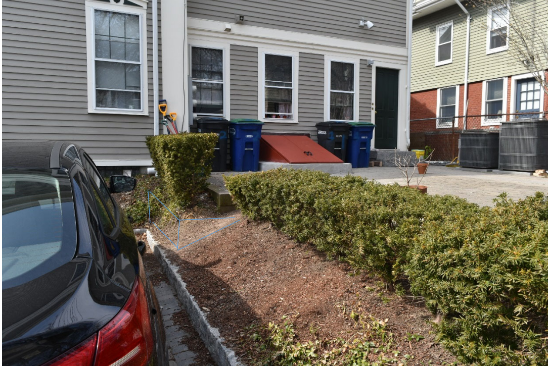
Steep slope near apartment patio to be retained with 3'6" x 2'6" L shaped pressure treated lumber cribbing adjacent to the cobble curb.
