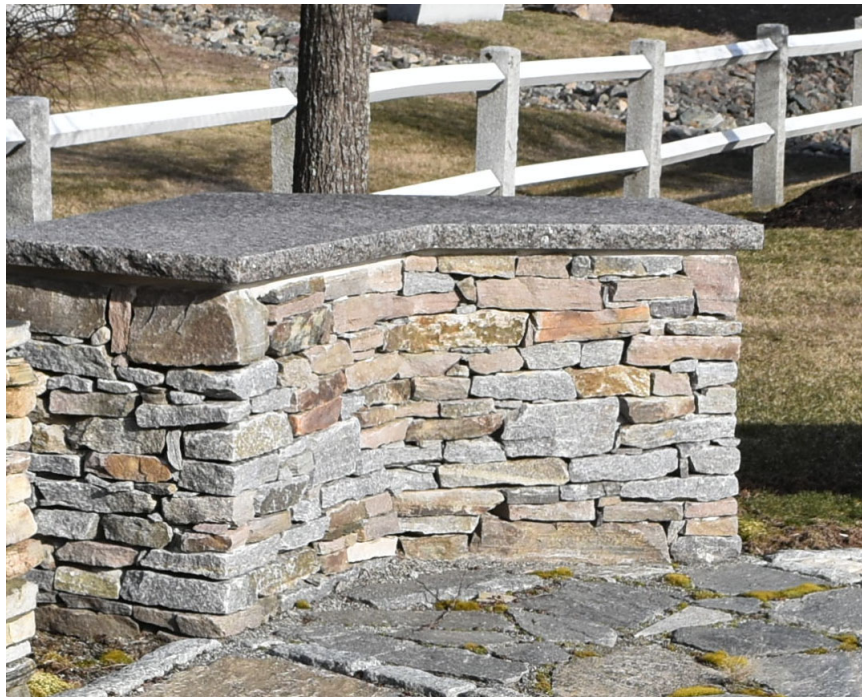
Example of Ticonderoga granite wall with bluestone cap- demonstration wall at Swenson Granite Works, Rowley, MA.
